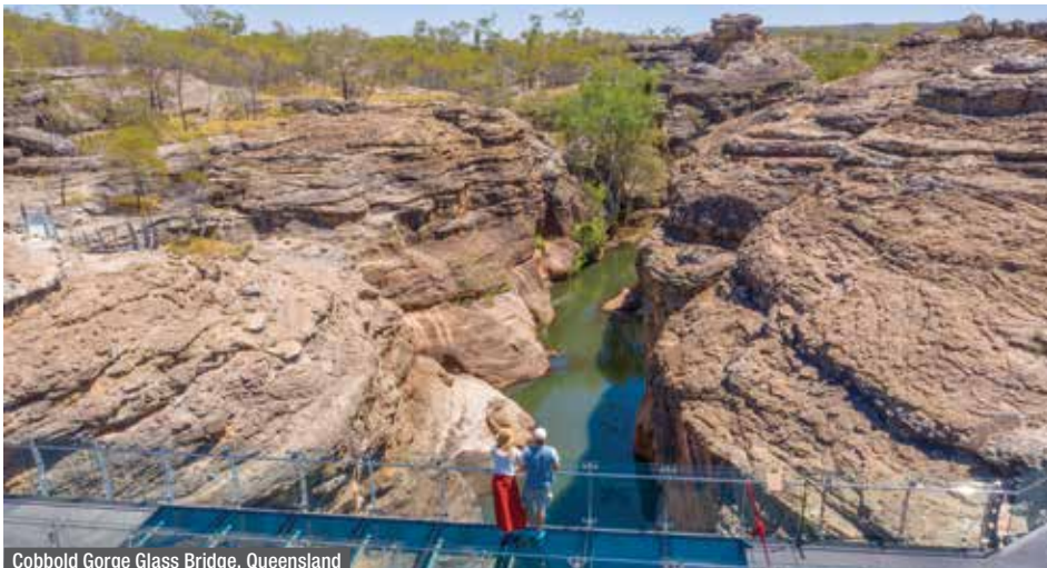
Cobbold Gorge Glass Bridge, Queensland
